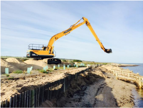
Figure 7 Beach renourishment and coir log installation
