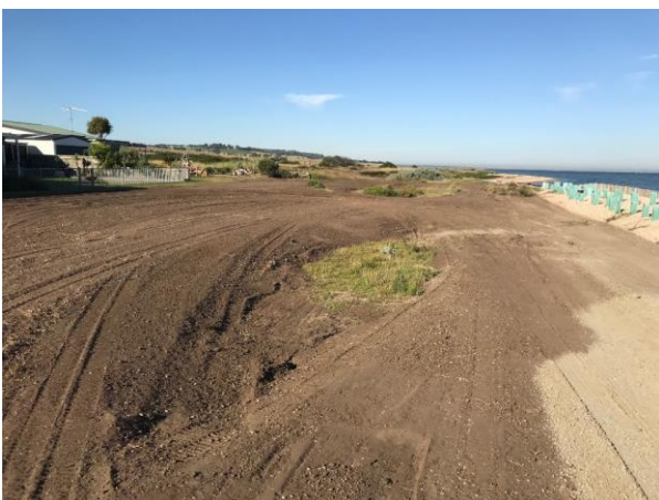
Figure 8 Onshore works - raising the level of the foreshore
